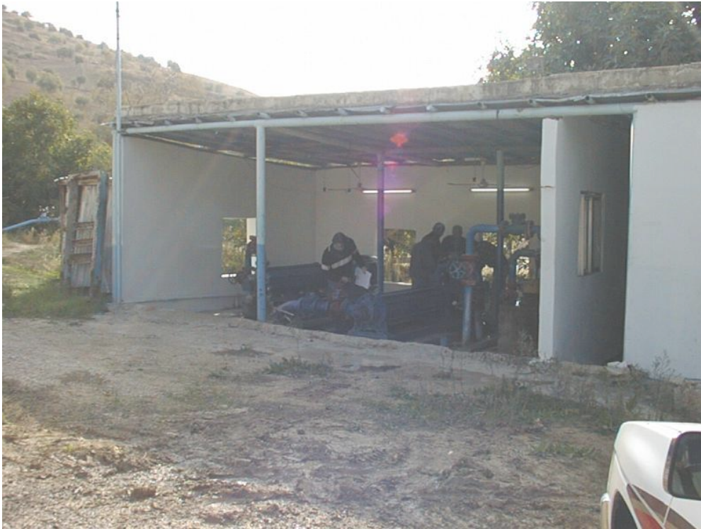
Figure 7: Judayta pumping station
