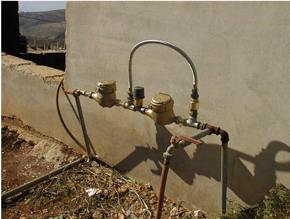
Figure 16: Air Release Valve Installation
